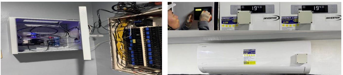
Fig 9. Visual Installation of the SBMS Device
